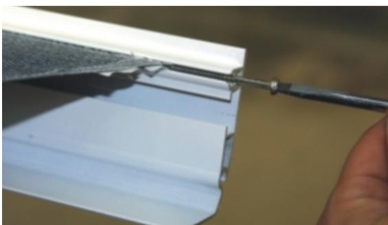
**3.-** Remove the 4x50mm screw, and replace it with a 4x70mm screw (available upon request Item No. 92114-490), tighten the screw to pull the fabric taut
